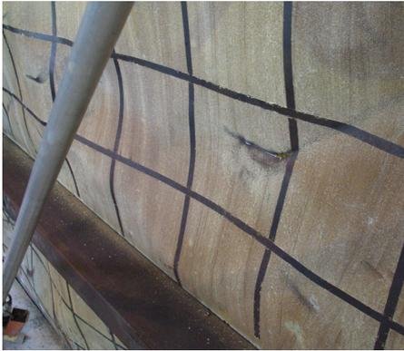
Photo 3. Steel plate crack.
